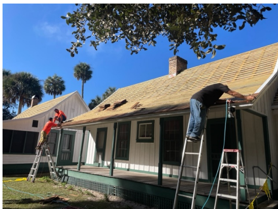
Roofers replacing the cedar shake shingles on Marjorie's house
