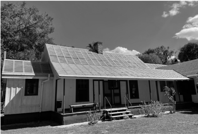
Re-roofing in progress
